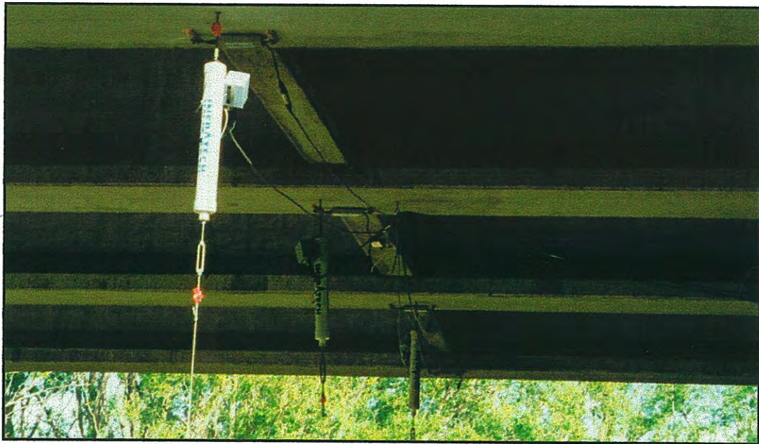
Figure 4.2 Instrumentation on the midspan of Waipara Bridge.
