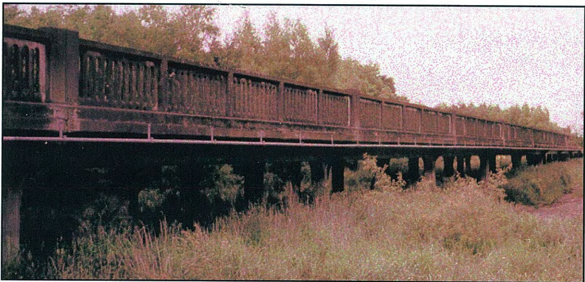
Figure 3.1 Rakaia Bridge, Canterbury, South Island, New Zealand.
