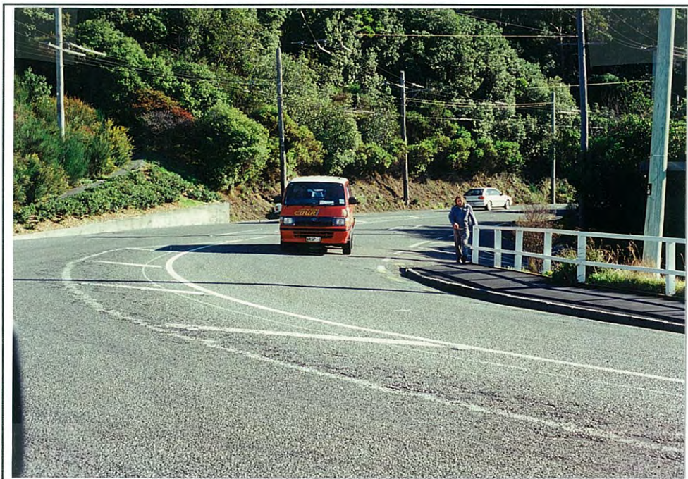
Figure 6.5 Overview of the Crawford Road bend, Wellington.
