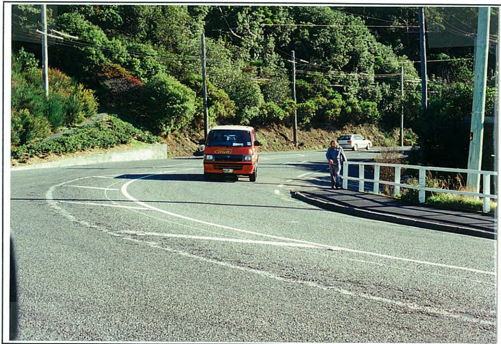
Figure 6.5 Overview of the Crawford Road bend, Wellington.
