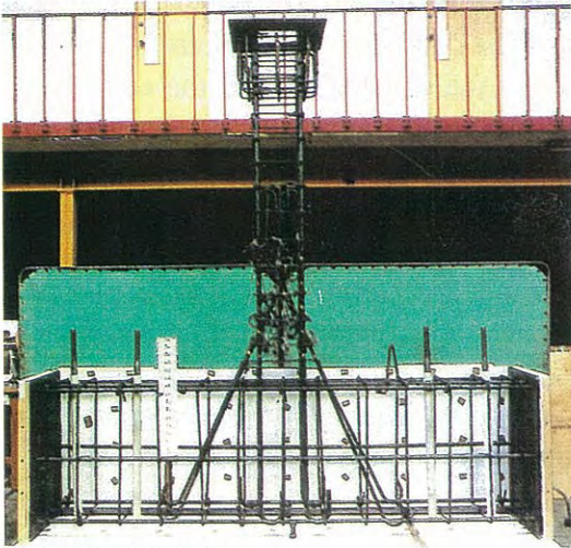
(a) Reinforcing steel cage
