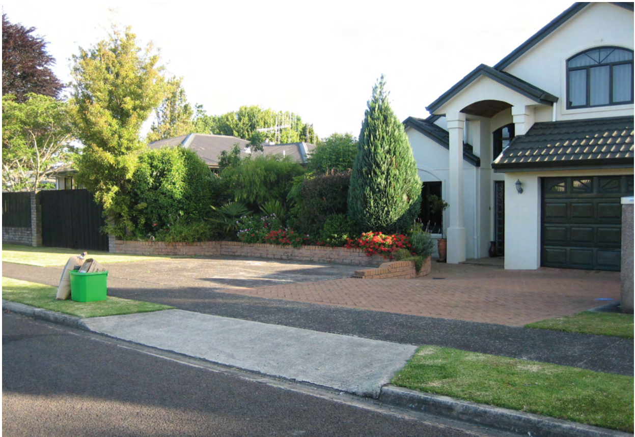
Photo 6.7 – Footpath continues to a high standard across driveway, Tauranga (Photo: Mike Calvert)
