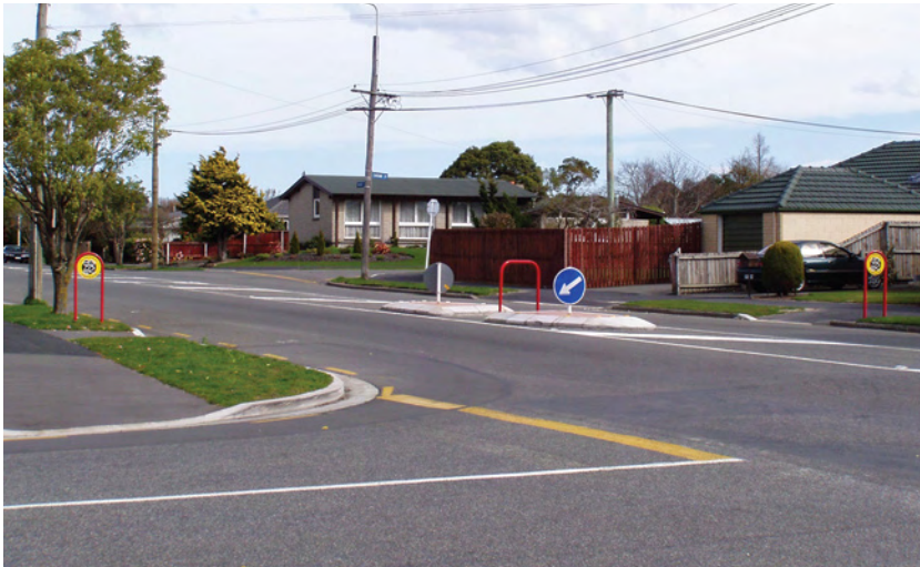
Photo 6.14 – Traffic island installed for safe routes to school, Christchurch (Photo: Tim Hughes)
