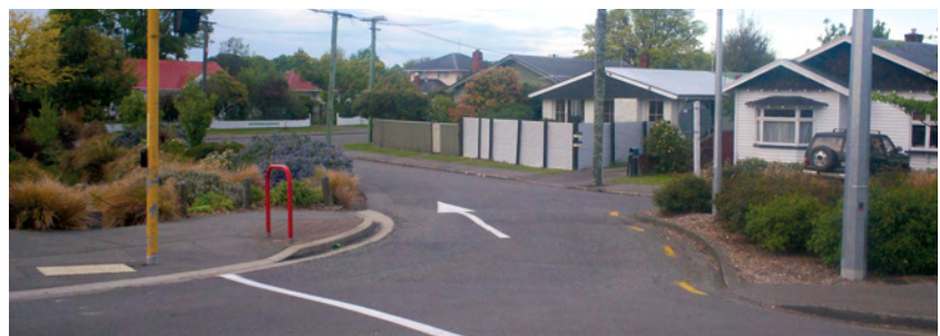
Photo 6.2 – Traffic reduction by one-way entry, Christchurch (Photo: Megan Fowler)
