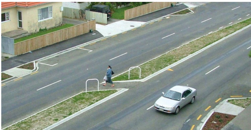
Photo 6.19 – Raised median with pedestrian cut-through, Palmerston North (Photo: Shane Turner) (note: tactile paving is missing)
