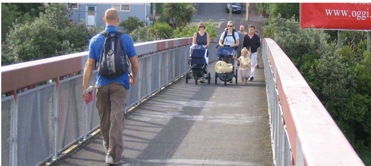
Photo 6.27 – Pedestrian overpass, Auckland (Photo: David Croft)
