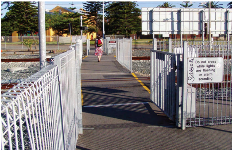
Photo 6.34 – Automatic pedestrian gates control double track crossing, Fremantle, Western Australia (Photo: Tim Hughes)
