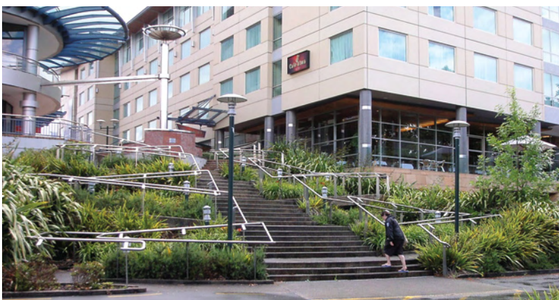
Photo 6.6 – Steps and zig-zag ramp, Hamilton (Photo: Shane Turner)
