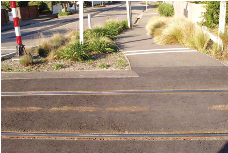
Photo 6.33 – Pedestrian railway level crossing beside road, Christchurch (Photo: Susan Cambridge)
