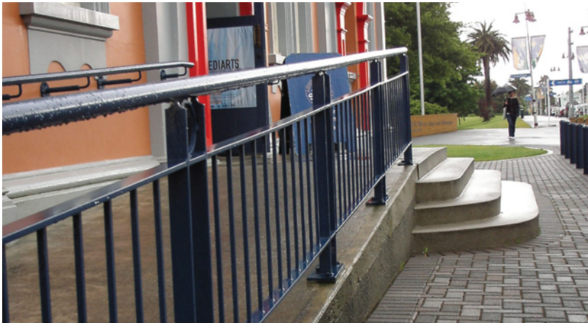
Photo 16.5 – Pedestrian fence, Hamilton (Photo: Shane Turner)
