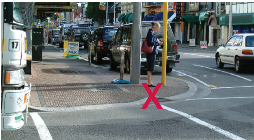
Photo 15.16 – Short kerb between crossing points is a tripping hazard, Christchurch (Photo: Paul Durdin)
