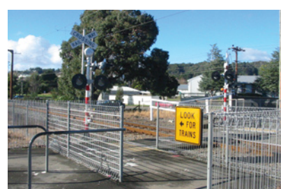
Photo 15.24 – Pedestrian rail crossing maze, Upper Hutt (Photo: Roy Percival)
