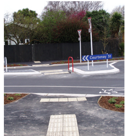
Photo 15.18 – Crossing point by roundabout, St Albans, Christchurch (Photo: Tim Hughes)
