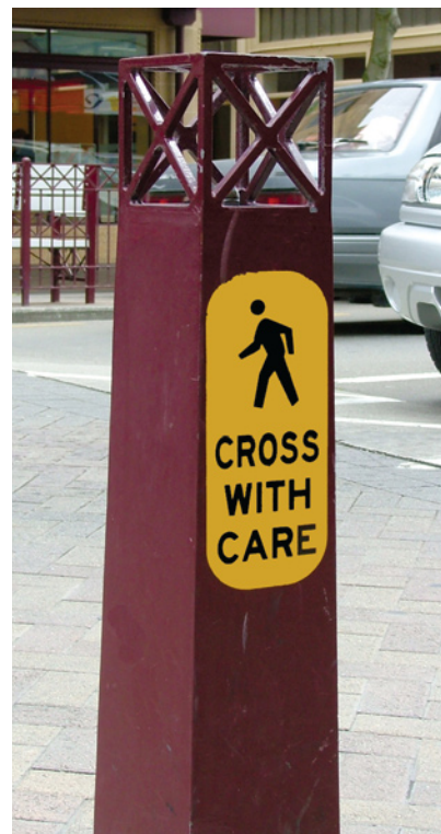
Photo 15.10 – Sign on bollard delineates edge of roadway, Palmerston North (Photo: Tim Hughes)
