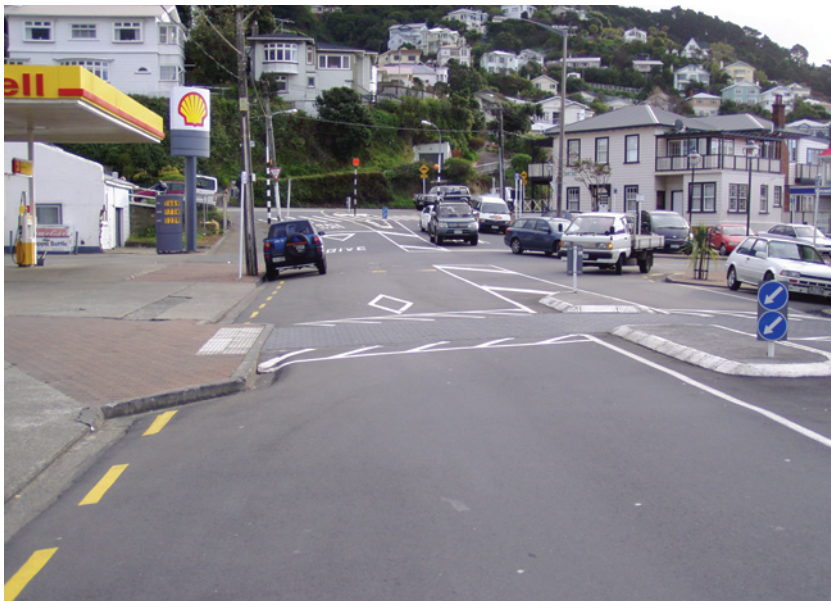
Photo 15.9 – Platform with good footpath to road contrast, Kilbirnie, Wellington (Photo: Tim Hughes)
