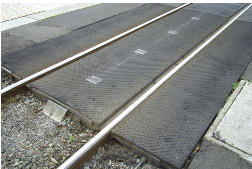
Photo 15.27 – Rubber crossing surface, Tauranga (Photo: Greg Hackett)
