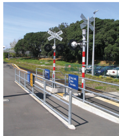
Photo 15.21 – Warning systems, Papakura (Photo: David Croft)
