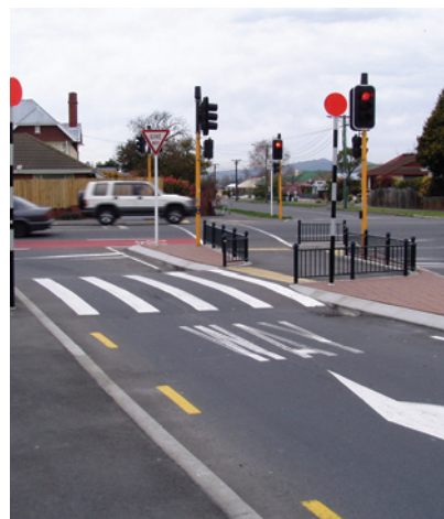
Photo 15.17 – Platform pedestrian crossing free turn, Northlands mall exit, Christchurch (Photo: Tim Hughes)
