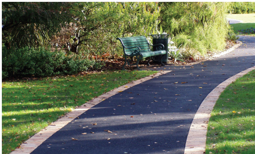
Photo 14.6 – Brick-lined asphalt path, Nelson (Photo: Tim Hughes)
