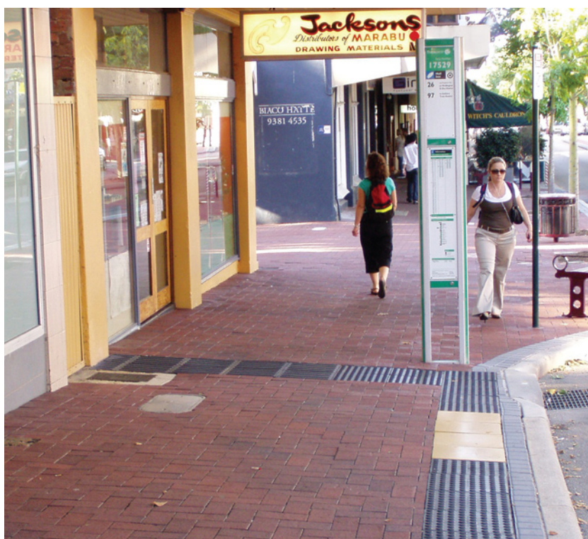
Photo 14.25 – Bus stop, with tactile pavement arrangement, Subiaco, Perth, Western Australia (Photo: Tim Hughes)
