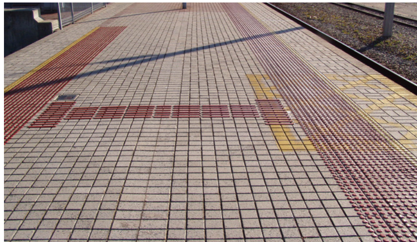
Photo 14.28 – Tactile paving treatment at railway station, Fremantle, Western Australia (Photo: Tim Hughes)
