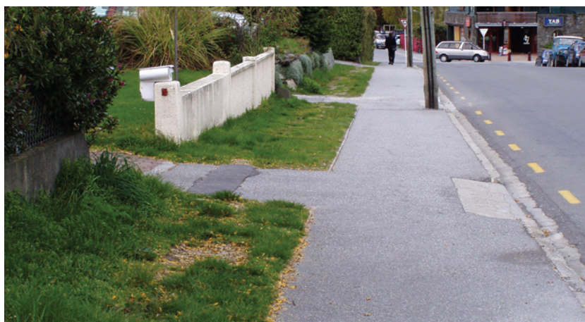
Photo 14.19 – Driveway with normal pedestrian path crossfall maintained, Queenstown (Photo: Tim Hughes)
