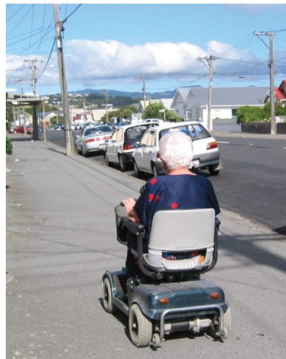
Photo 14.5 – Footpath with acceptable crossfall, Wellington (Photo: Lesley Regan)
