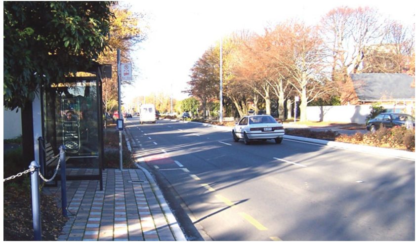
Photo 14.26 – Bus shelter in street furniture zone (through route behind shelter), Christchurch (Photo: Aaron Roozenburg)
