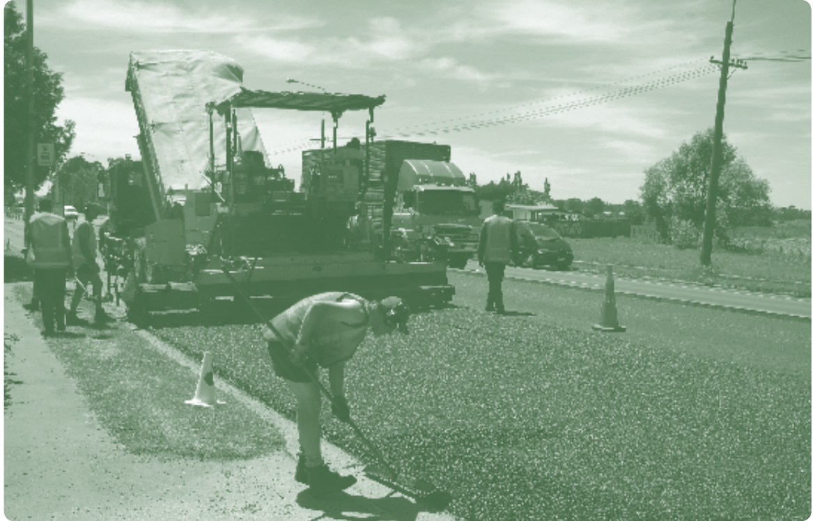
Laying down asphalt
