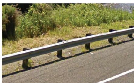
b) Semi-rigid W-beam barrier
