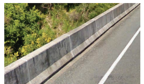
c) Rigid concrete barrier (segmental system)
