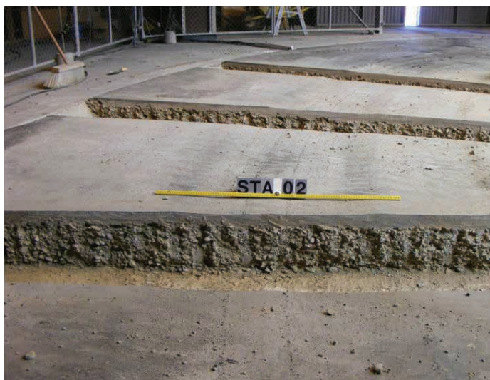
Test 2 example from the Canterbury Accelerated Pavement Testing Indoor Facility (CAPTIF)
