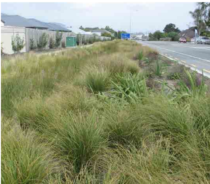
Roadside swale of tussock sedges, rushes and mountain flax filtering road runoff, Stoke, Nelson.
