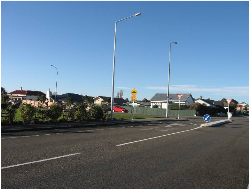
Photo 6. One of the projects implemented, which included vegetation spreading at centre left and speed platform centre right. The vegetation intentionally obscures visibility leading up to the intersection. This coupled with the speed platform forces vehicles to slow.
