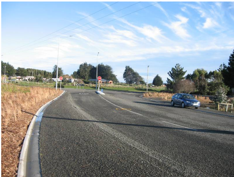
Photo 7. Chesney/Scott Street Intersection which was 'Teed – up'; a physical outcome of the NAPS programme.
