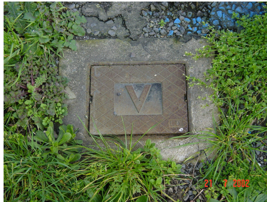
Typical Toby Box Installation
