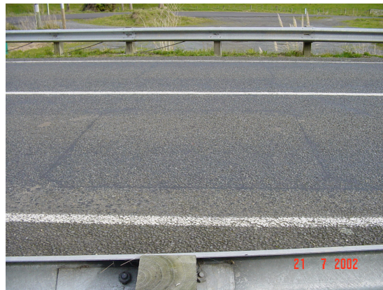
Typical Completed Loop
