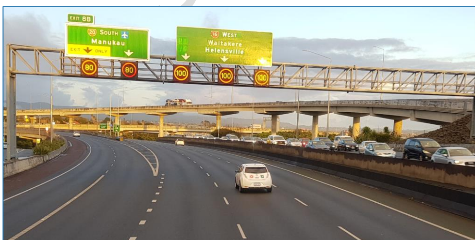
Figure 8. LCSs on a gantry spanning motorway
