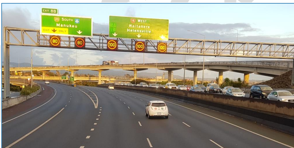
Figure 5. LCS on a gantry spanning motorway
