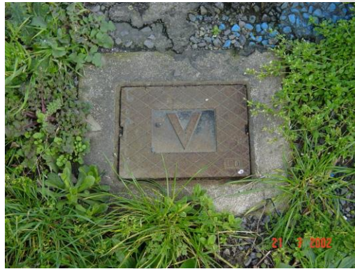
Typical Toby Box Installation
