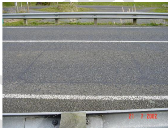
Typical Completed Loop
