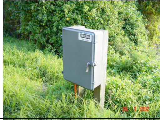
Typical Harding 2002 Cabinet Typical Montrose Cabinet Continuously Powered Sites Non - Continuously Powered Sites
