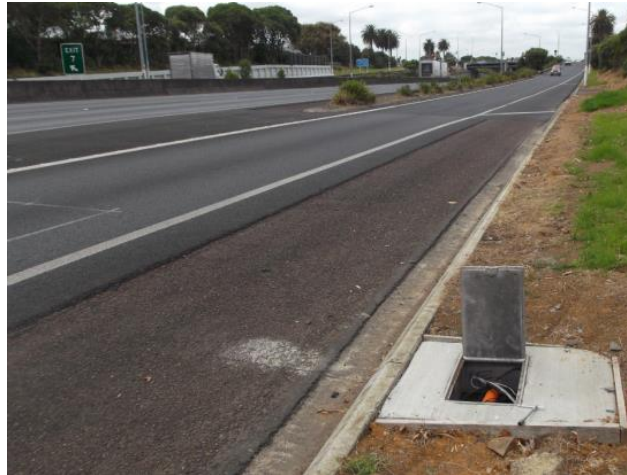
Figures 8 and 9. A purpose-designed cable jointing box has been designed and strength tested for use on the network.
