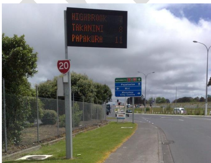
Figure 11. Type D/EJT sign installed over the footpath. This sign was damaged by large vehicles exiting the industrial site on the left — the swept path of heavy vehicles can be seen on the footpath.
