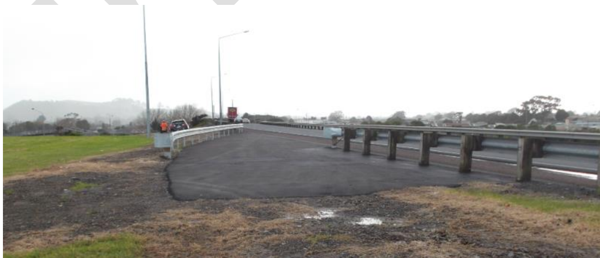
Figure 18. New maintenance access for CCTV site that doubles as a grass-cutting maintenance access site.
