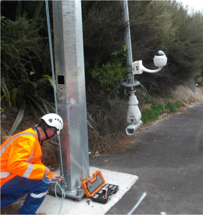
Figure 3. Safe CCTV camera maintenance at ground level.
