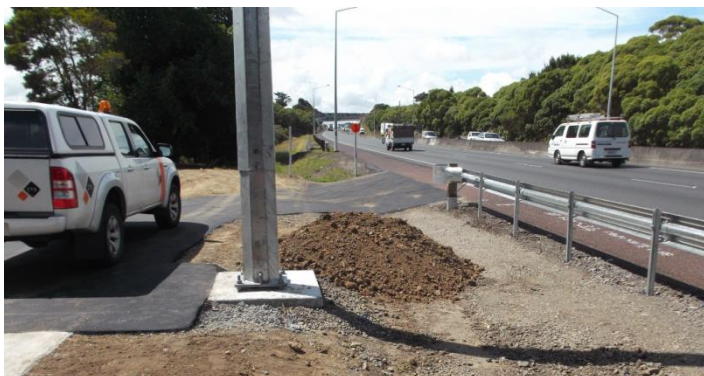
Figure 15. Maintenance access under construction with asphalt surface and barrier protection.
