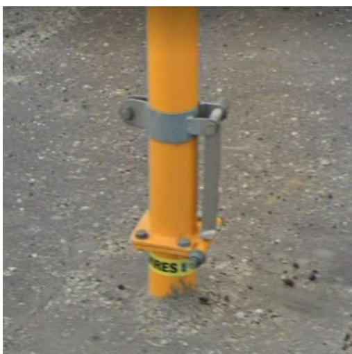
Figure 1. Typical bracket to support weight and enable pole to be lowered without resting on the signal aspects or equipment
