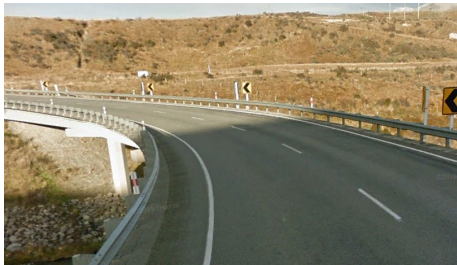
Metal barrier within 5m of edgeline
