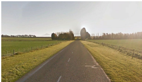
Frangible posts or level and safe slopes ( \leq 15 degrees and \leq 1 m high) within 5m of edge of seal (no edgeline)
