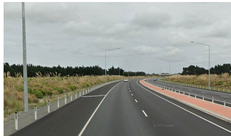
Wire rope barrier within 5m of edgeline
