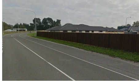
Semi-rigid structure (timber fence) 5–10m from edgeline
