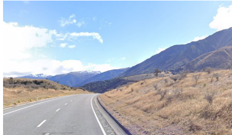
Upslopes (> 15 degrees and > 1m height difference) within 5m of edgeline
