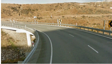
Metal barrier within 5m of edgeline
