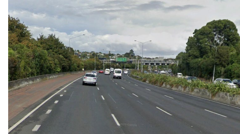
Concrete barrier within 5m of edgeline
