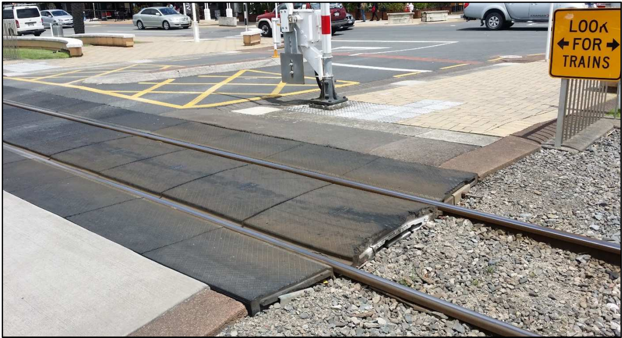
Figure 33: Rubber panel crossing treatment for road and path (CBD, Tauranga)
