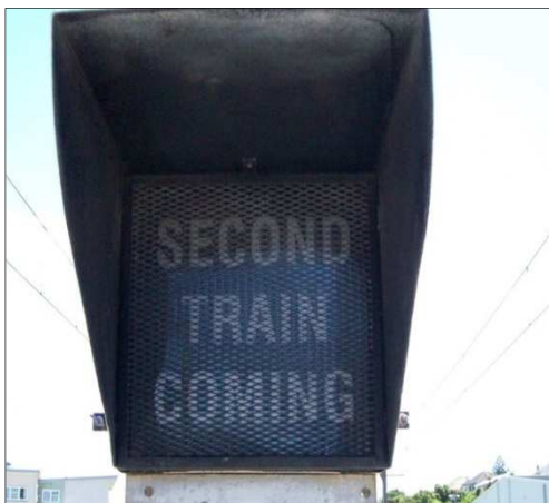
Figure 30: Example of an active warning sign
