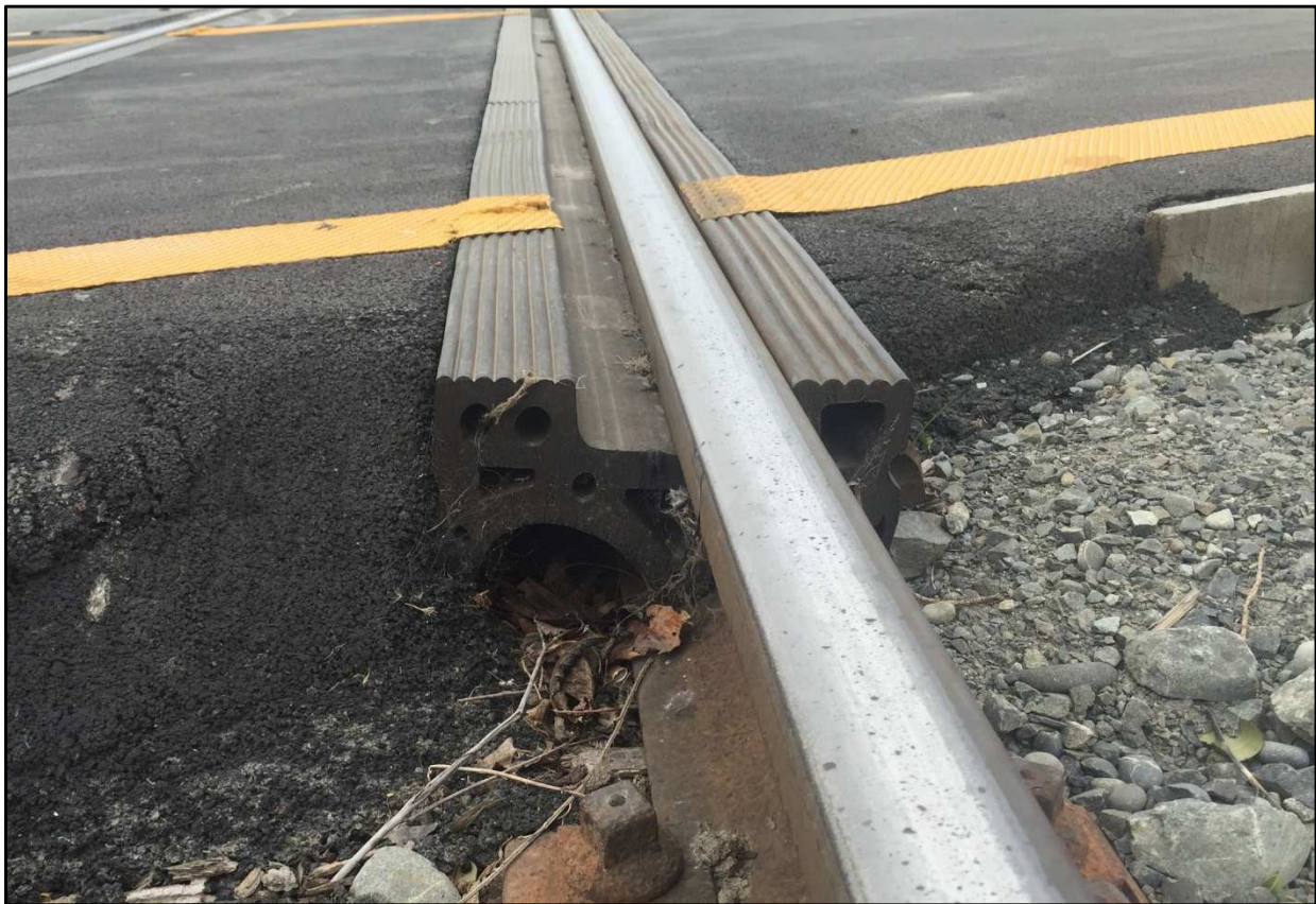
Figure 34: Epflex railseal used on asphalt railway level crossing (Kaiapoi)
