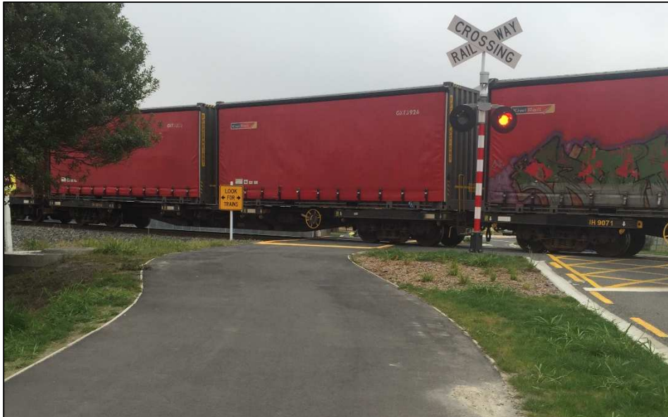
Figure 43: Flashing lights and bells on a path approach (Kaiapoi)
