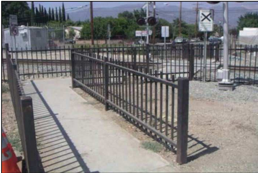
Figure 44: Example of a Z-crossing approach, albeit too narrow for easy cycle use (FRA 2016)
