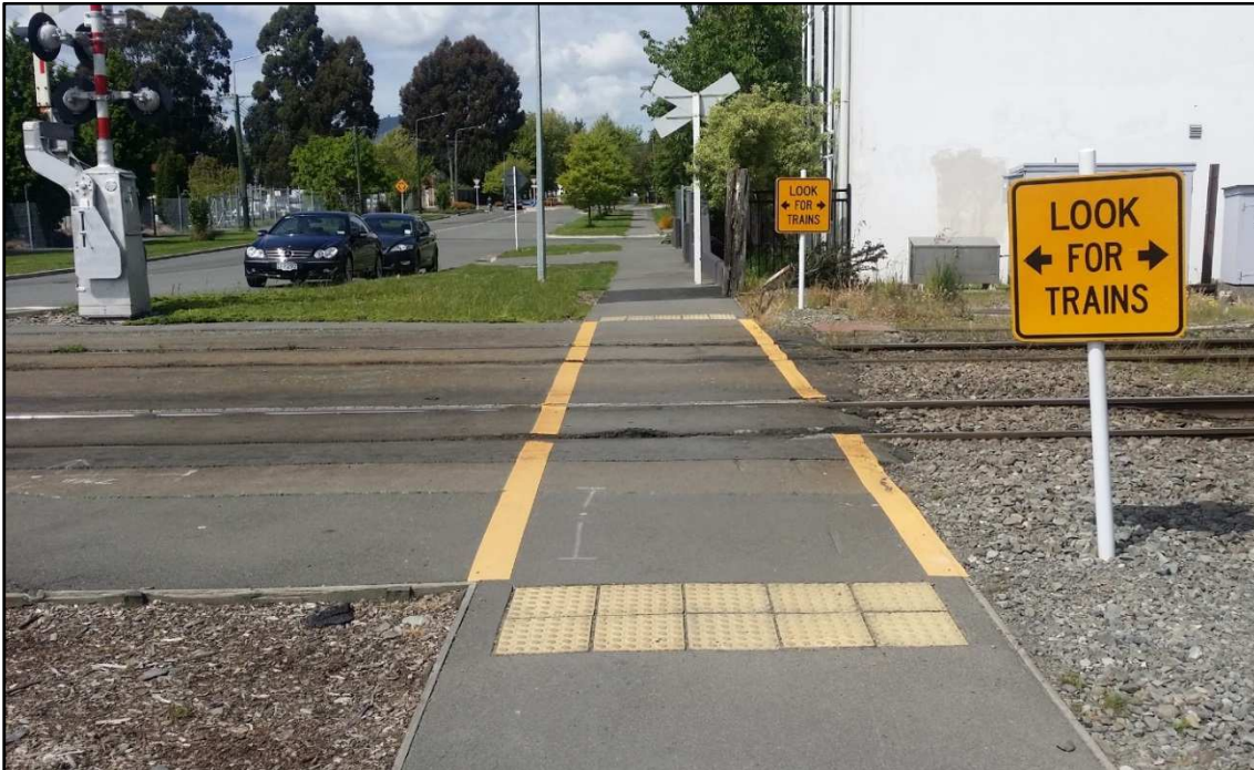
Figure 24: TGSIs at level crossing - note no limit line applied (Grove Road, Christchurch)
