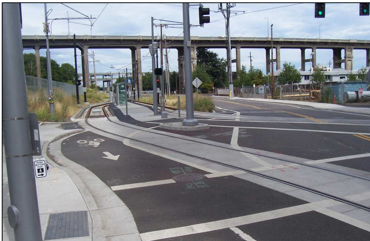
Figure 14: A cycle lane is re-aligned to cross a railway closer to 90 degrees (Portland, OR, US)
