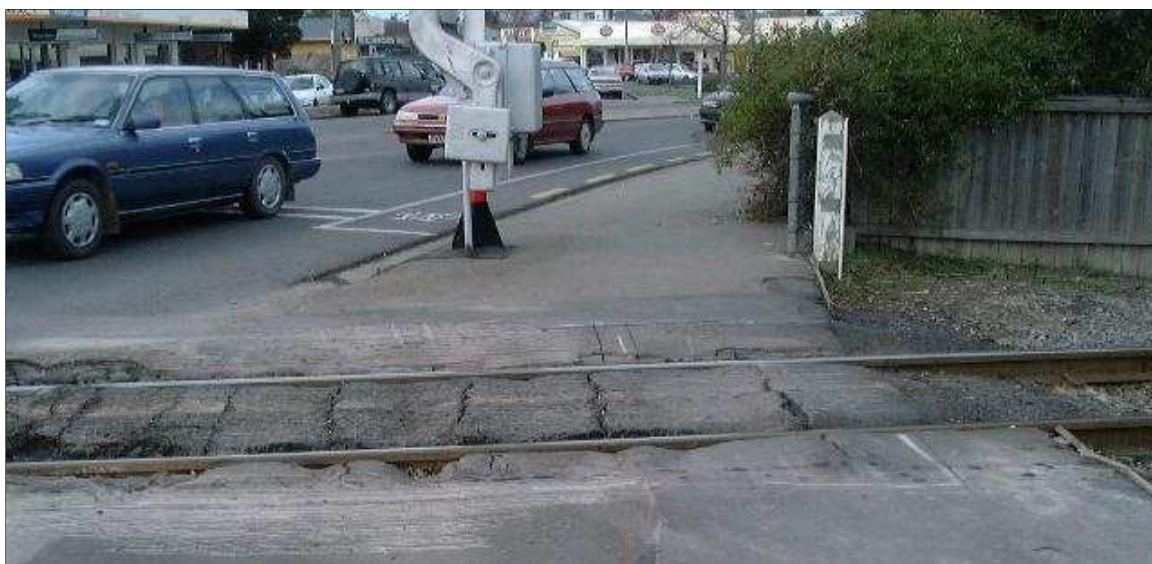
Figure 32: Poor pathway maintenance affects the safe available path for many users
