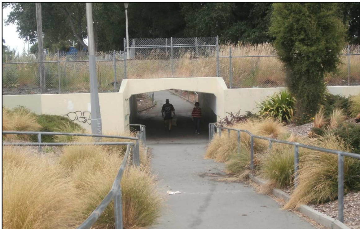
Figure 40: Railway underpass at Kyle Park with good sight lines, Christchurch
