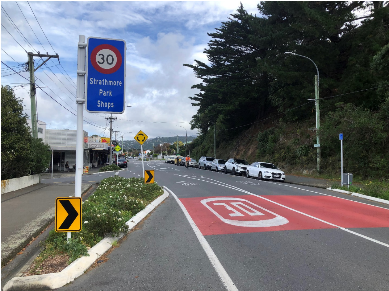
Figure 1 Coloured surfacing at a speed limit threshold (Photo: Ann-Marie Head)
