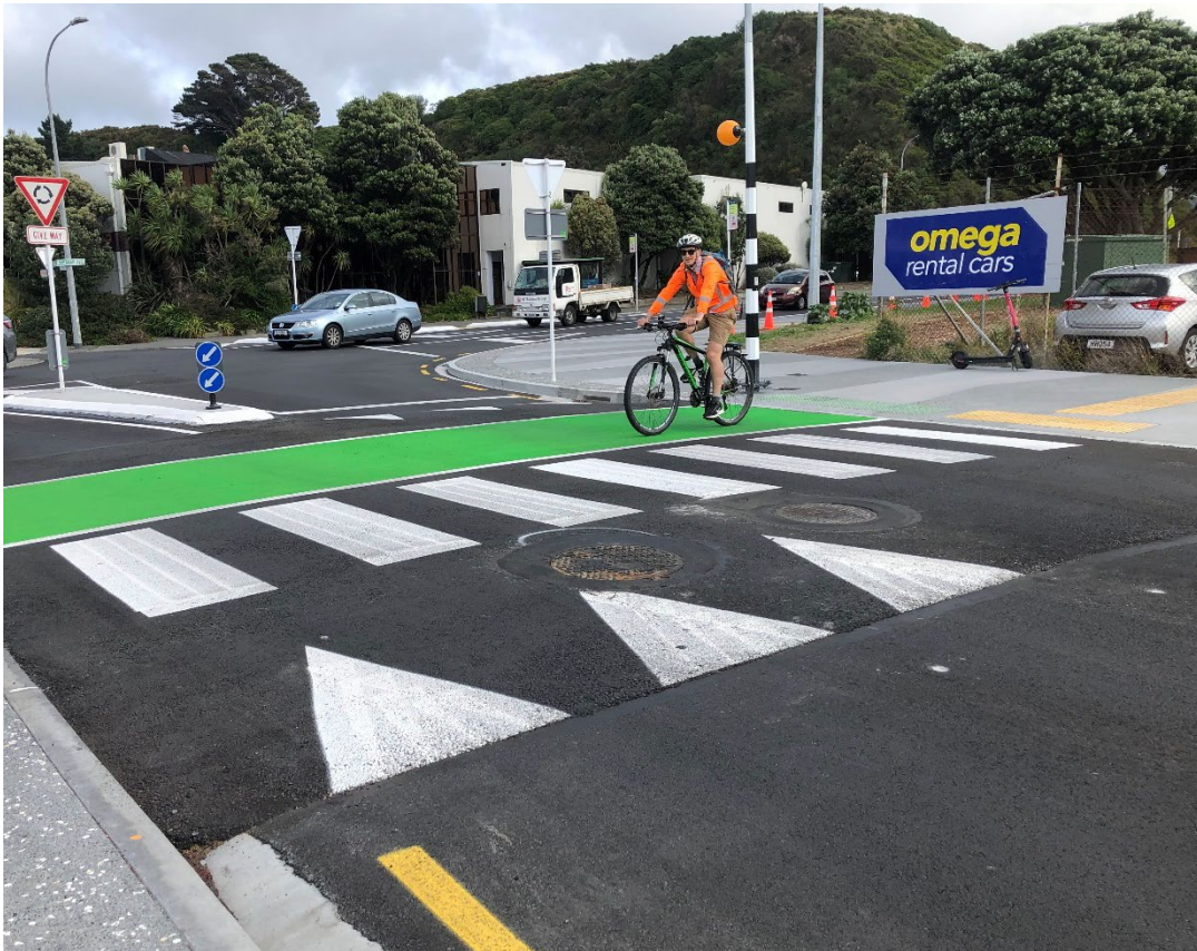
Figure 3 Application of green surfacing on a cycle crossing (Photo: Ann-Marie Head)
