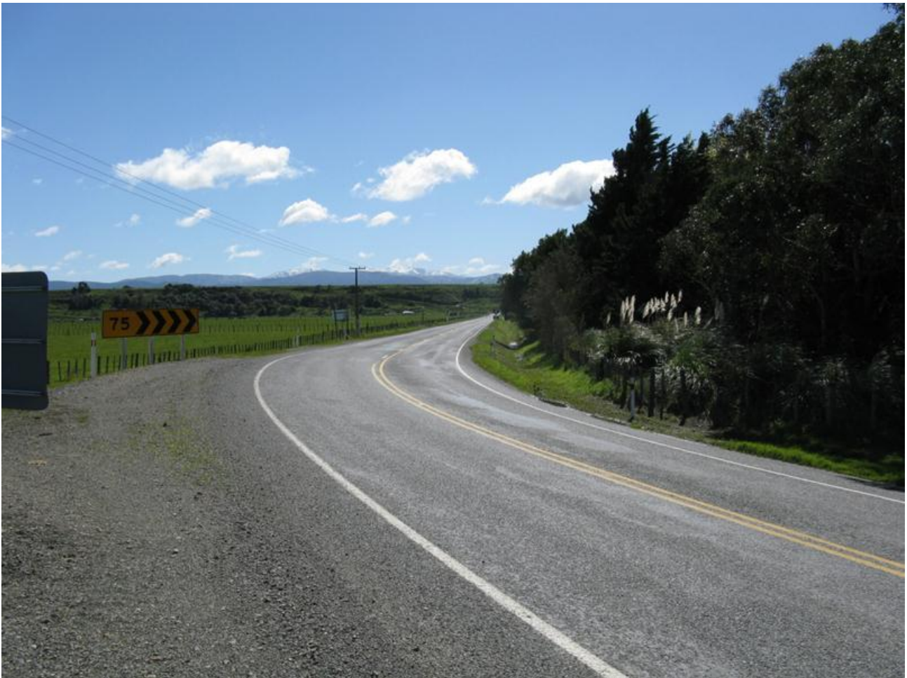
Figure 17: Corner F (SH53 RP0/0 13990-14080) (decreasing direction is from bottom to top)
