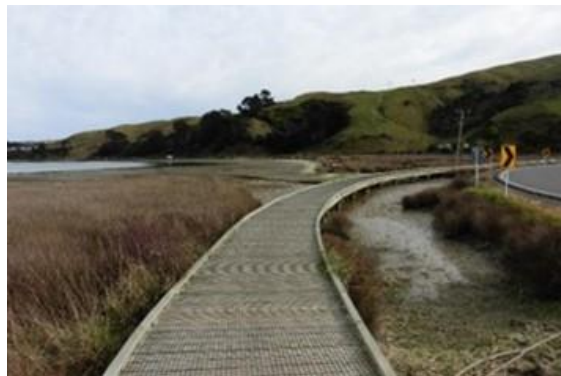
Edge treatment provided on a boardwalk with no fence or barrier. Pauahatanui Estuary boardwalk (photo: James Wratt)
