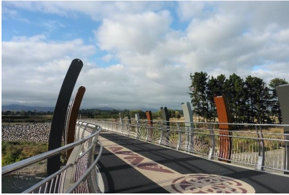
Both a hand rail and deflection rail prevent handlebars from snagging the vertical barrier elements. He Ara Kotahi, Manawatu River bridge (photo: James Wratt)
