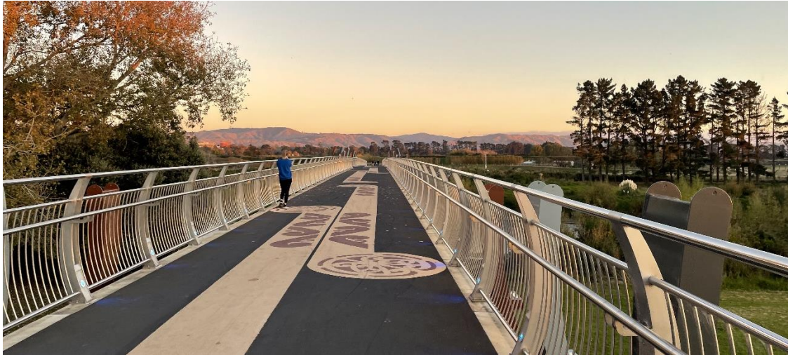
A taller fence may improve perceived safety for people cycling and walking. Manawatū River bridge, He Ara Kotahi (photo: James Wratt)
