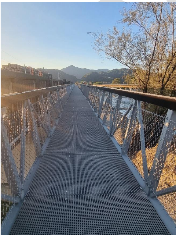
Outward leaning fence on a narrow bridge increases useable width for cyclists. Wairau River Bridge, Marlborough (photo: Peter Kortegast).
