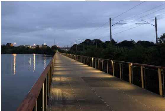
1200mm fence where risk of angled collision is low. Orakei Basin Boardwalk, Auckland
