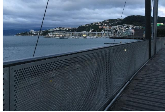
Perforated panels prevent handlebars and bicycle wheels from being trapped or catching in the fence. Whairepo Lagoon Bridge, Wellington Waterfront (photo: James Wratt)
