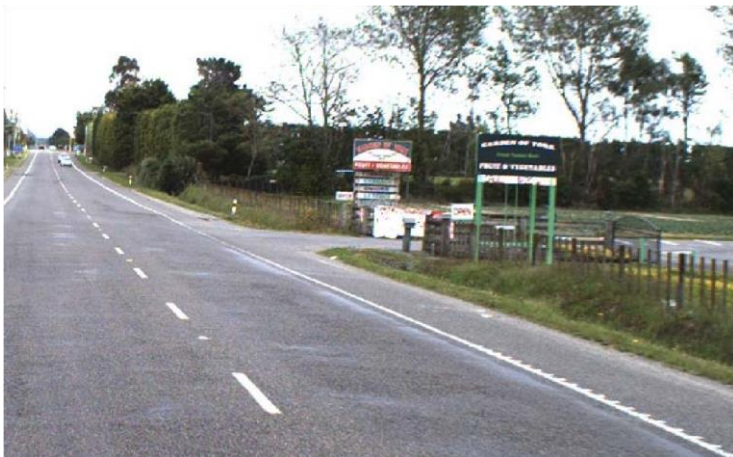
Figure 6-2: Continuity of edgeline ATPM broken at an access point
