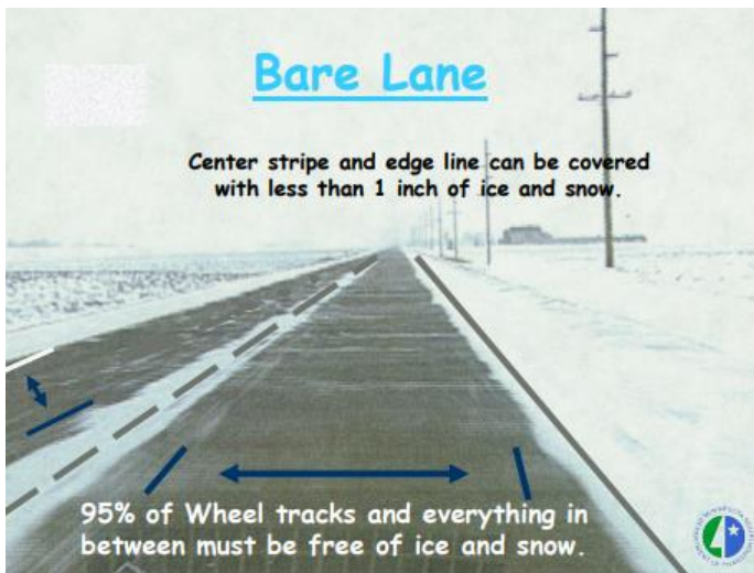
Figure 6-4: Example of Bare Lane Roadway Condition from the Minnesota Department of Transport
