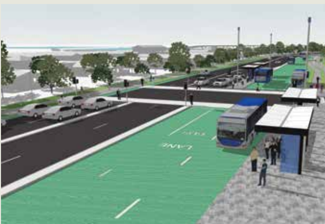
PAKURANGA ROAD BUSWAY - PART OF THE PROPOSED BUSWAY FROM PANMURE TO PAKURANGA. BUS STOPS ARE AT INTERSECTIONS TO IMPROVE SAFETY FOR PEDESTRIANS.
