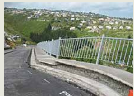
DAMAGE FROM THE FEBRUARY 2011 EARTHQUAKE - ROTATED GABION BASKET RETAINING WALL, GLENSTRAE ROAD, REDCLIFFS, CHRISTCHURCH.
