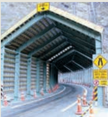
TEMPORARY PORTAL AT THE ENTRANCE TO THE HOMER TUNNEL
