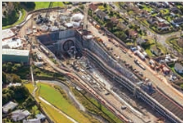
SOUTHERN APPROACH TRENCH OF THE WATERVIEW CONNECTION PROJECT
