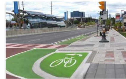
Cycle, footpath and pedestrian crossing facilities alongside the Viva BRT system
