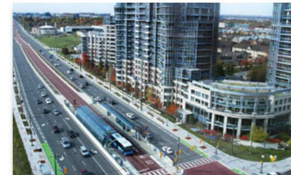
Development along the Viva BRT corridor
