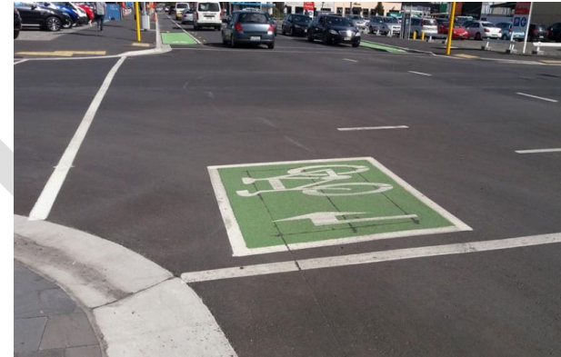
Figure 24: A hook-turn box on a flat surface with space for manoeuvring around it in Christchurch (Jeanette Ward)
