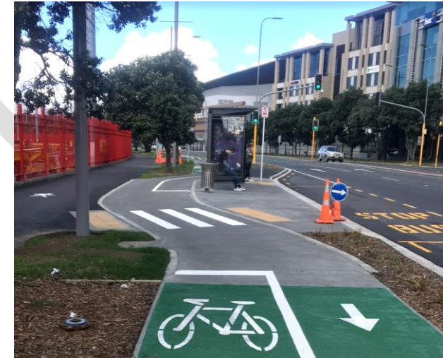
Figure 26: Bus stop bypass featuring clearly differentiated cycleway with clear markings and varied materials, appropriate geometry, tactile pavers, conspicuous crossing. Visibility could be improved if there were clear glass panels at both ends of the bus shelter. (Sam Hood, 2020)
