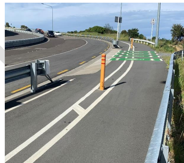
Figure 8: Appropriate bollard design, featuring a tall bollard with coloured reflective treatment, good sightlines, and clear delineation on approaches (NZ Transport Agency Waka Kotahi)
