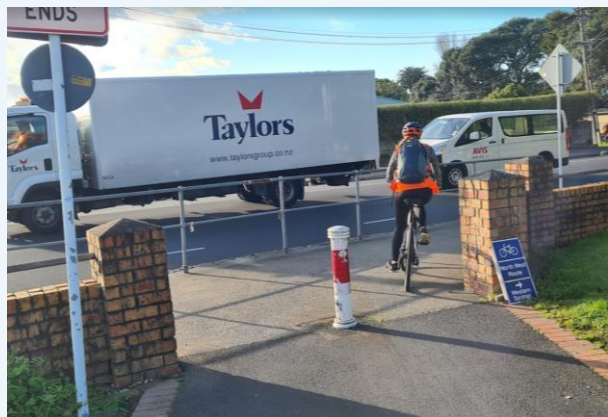
Figure 7: This bollard is unnecessary for motor vehicle access control and restricts manoeuvring space at a tight corner - North-western Cycleway, Carrington Road, Auckland (Sam Hood, 2022)
