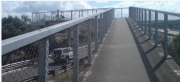
Figure 14: A motorway overbridge with a steep gradient – North-western Cycleway, Auckland (replaced with underpass since photo taken) (Bike Auckland, n.d.)
