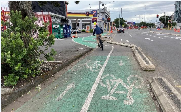
Figure 15: A problematic combination of having to navigate tight horizontal geometry and mounting of a ramp on an angle simultaneously on Quay St, Auckland. (Lukas Adam, 2023)
