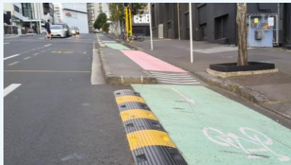
Figure 25: A bypass too narrow for some users (1.25m), with sharp grade changes. Victoria Street, Auckland. (Sam Hood, 2022)
