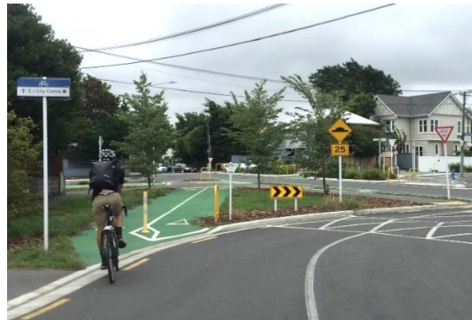
Figure 28: Clear and legible cycle wayfinding. Signage supports, rather than leads for legible design – intersection of Buccleugh St and Cashel St, Christchurch (Malcolm McCracken, 2022)
