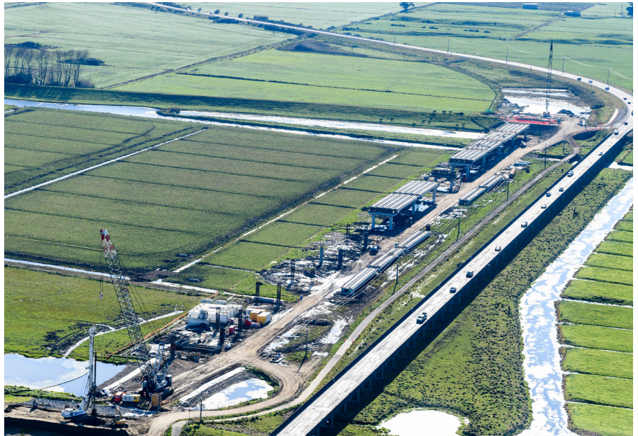
Whirokino Trestle Bridge
