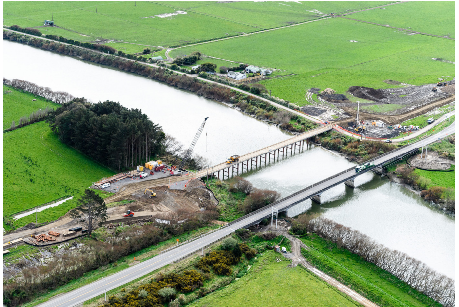
The Manawatū River Bridge and the temporary staging bridge
