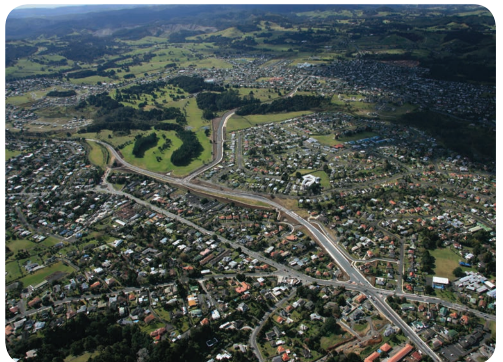
Under construction, August 2011
