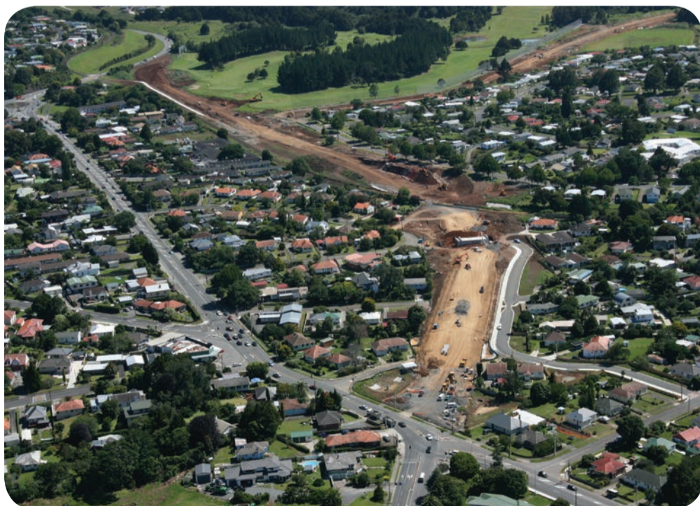
Under construction, January 2011
