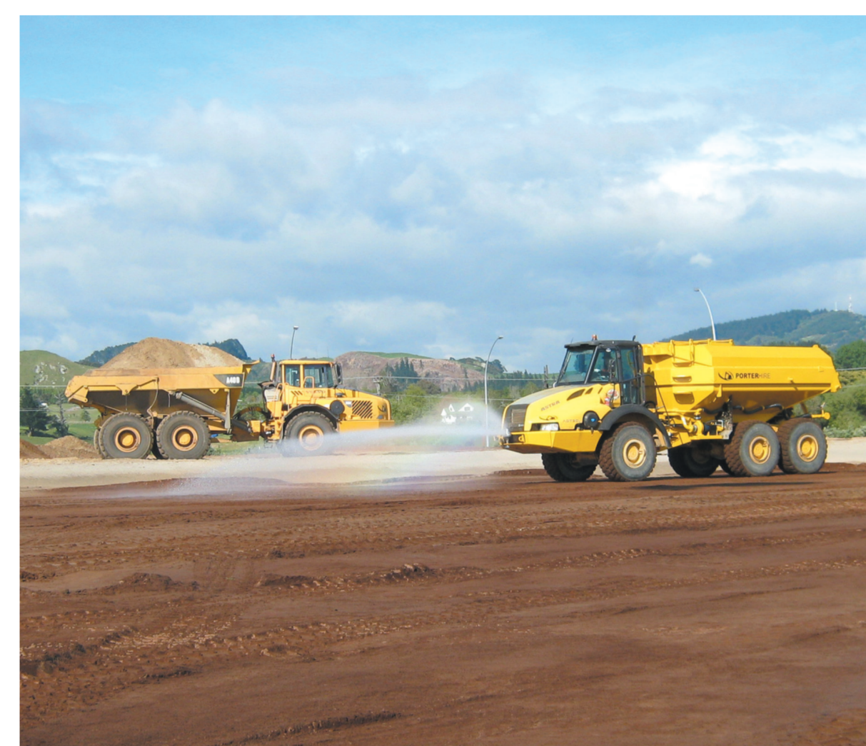
Water carts watering exposed ground
