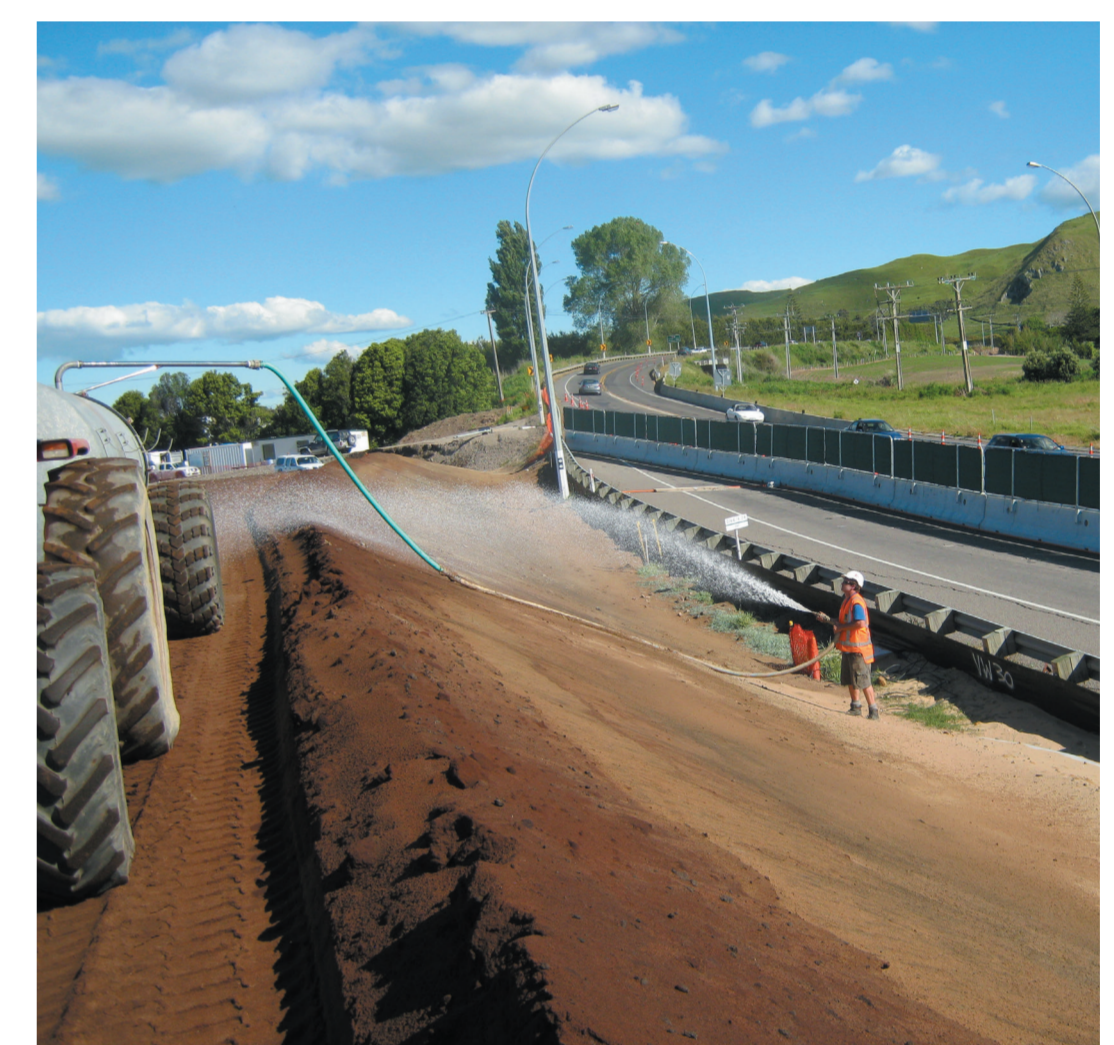
A dust suppressant is sprayed on to exposed dirt and sand, as it dries it forms a crust
