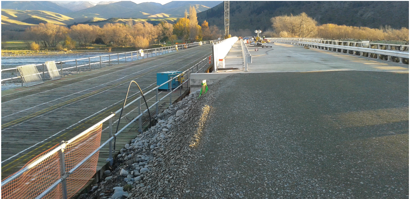
The new No 1 Bridge looking toward the Kurow township
