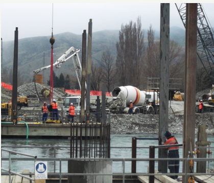
Work on Bridge 2 viewed from Kurow to Island.
