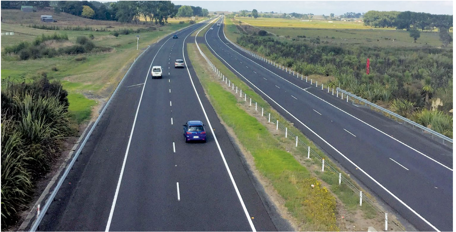
Rebuilding work on the lanes south of Kainui Road bridge start later this month
