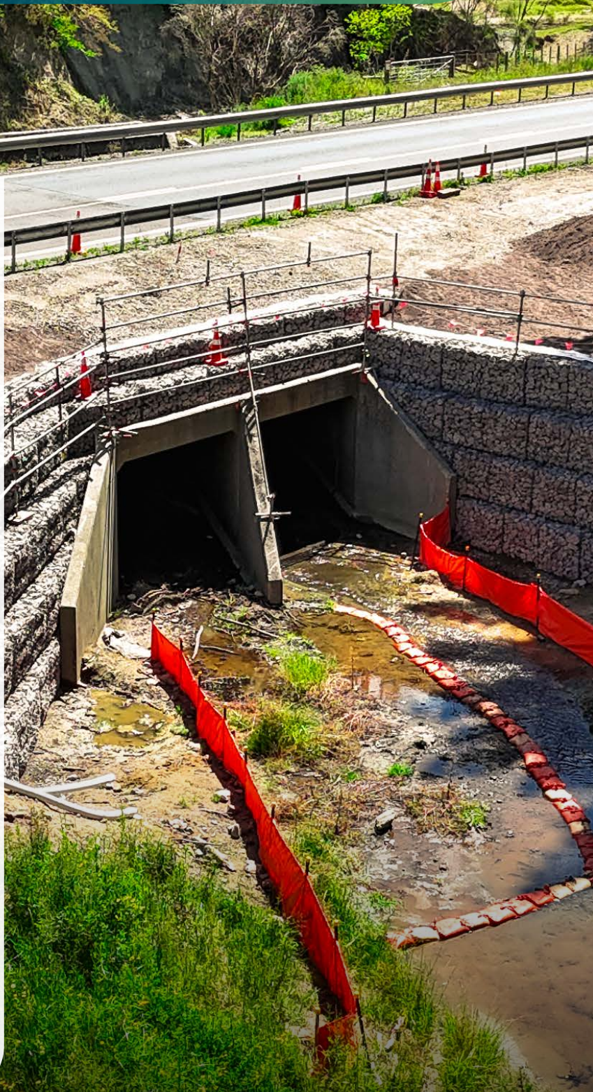
Dillon's Hill Culvert, State Highway 5
