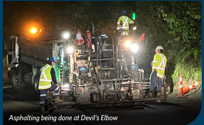
Night works at Devil's Elbow in July
