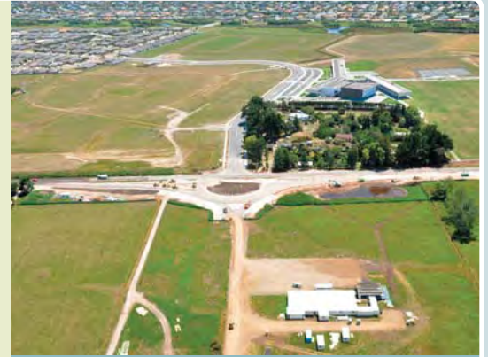
Tara Road site office and visitor information centre under construction, February 2011.
