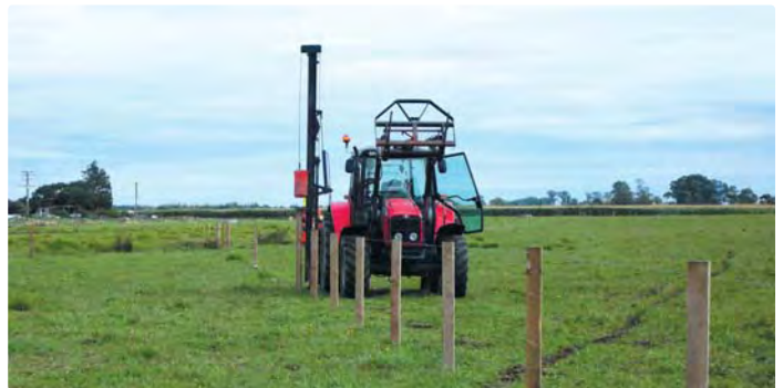
Preliminary work under way - fencing along Pah Road.
