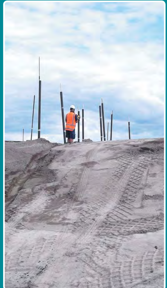
Tara Road trial embankment nearing completion.
