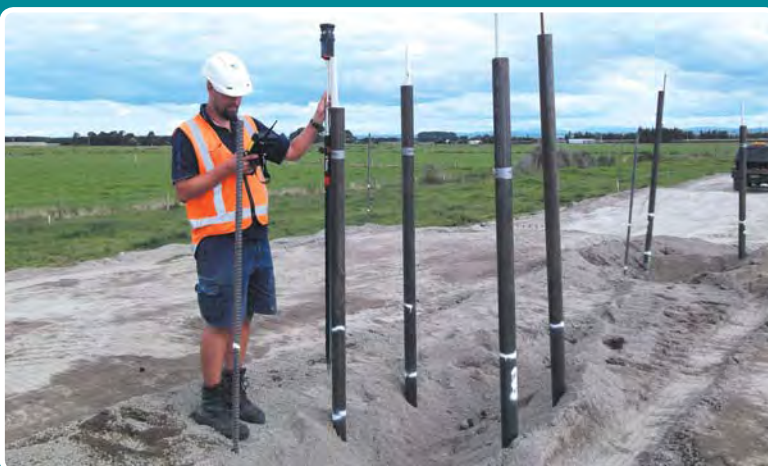
Surveyor monitoring the geotechnical equipment.
