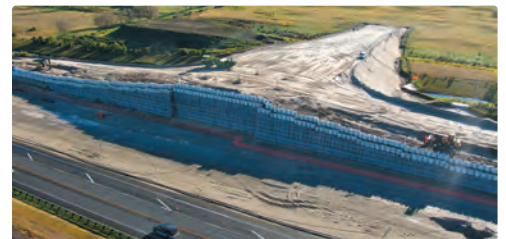
Mangatawa interchange MSE wall construction (beach side)
