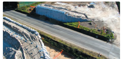
Maketu Road bridge MSE walls
