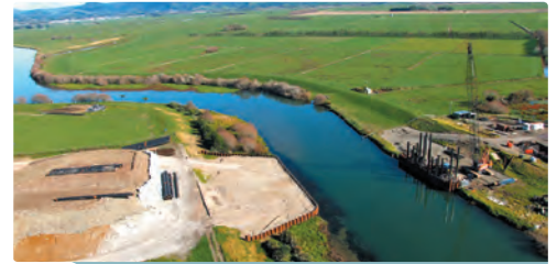
Kaituna River bridge
