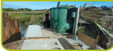
Diagonal drain pump station upgrade
