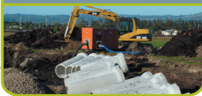
Parton Road bulk watermain relocation
