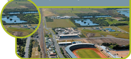
Maranui stormwater treatment pond enlargement
