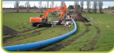
Mangatawa Lane to Domain Road bulk watermain relocation
