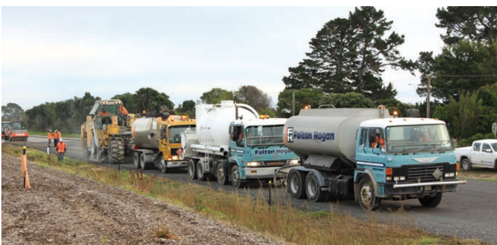
Foamed bitumen stabilisation of the base layer (Type B )
