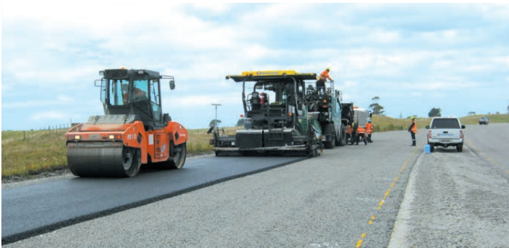
Asphaltic concrete being paved over chipseal (Type A )
