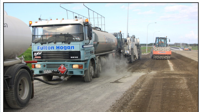
Above: Final 140,000m 2 (equivalent to 28 rugby fields) foamed bitumen stabilised base course—April 2015
