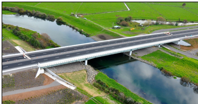
Above: Kaituna River bridge
