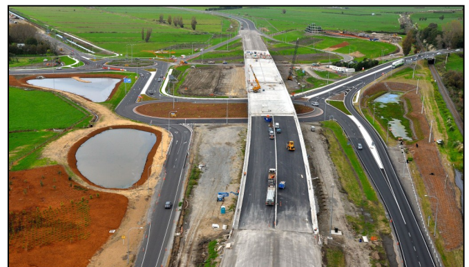
Above: Domain Road interchange
