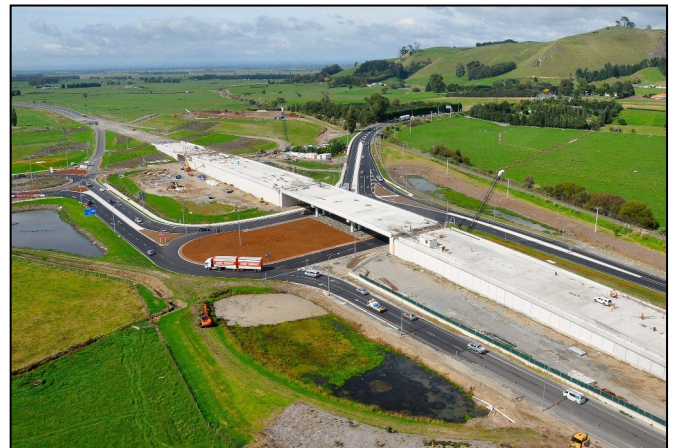
Above: Domain Road interchange
