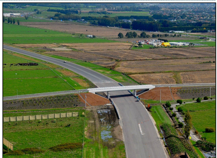
Above: April 2015—Parton Road bridge completed
