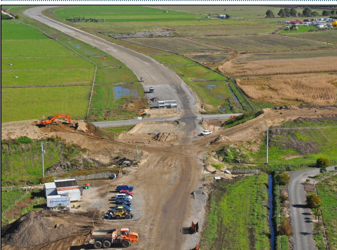
Above: April 2014—Parton Road bridge approaches
