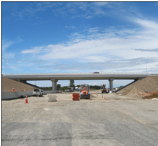
Above: Parton Road bridge
