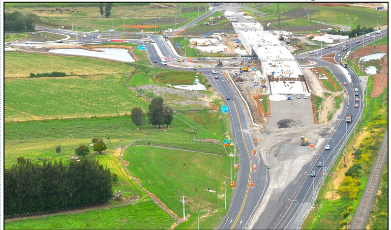
Below: SH2 / Domain Road interchange—Feb 2015
