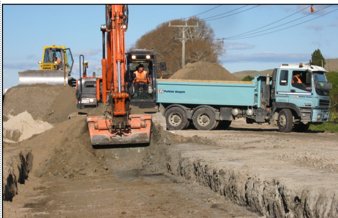
Above: Removal of the old State Highway 2 material and the placement of surcharge
