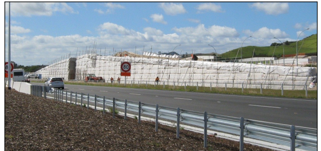
Above: Mangatawa Interchange central embankment
