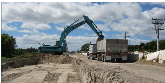
Above: Pavement box-cut operation near Bruce Road.
