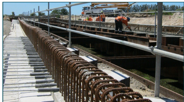
Left: Mowing Boat Culvert C.
