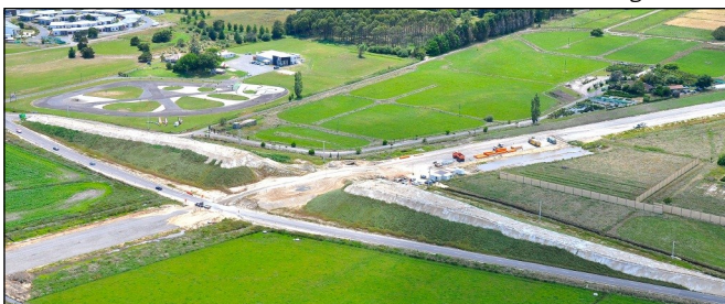
Below: Parton Road bridge site
