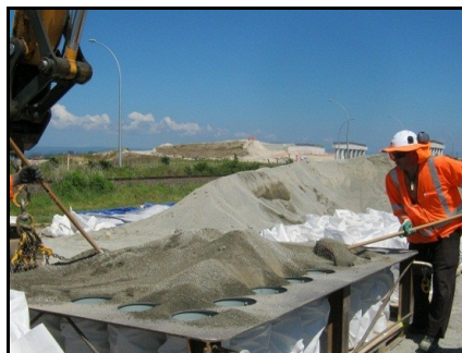
Above: Cement treated material fills the bags
